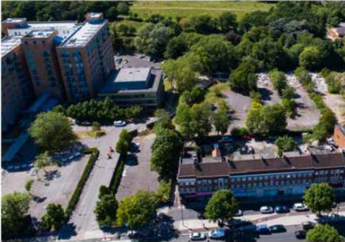
Aerial View of Existing Site
